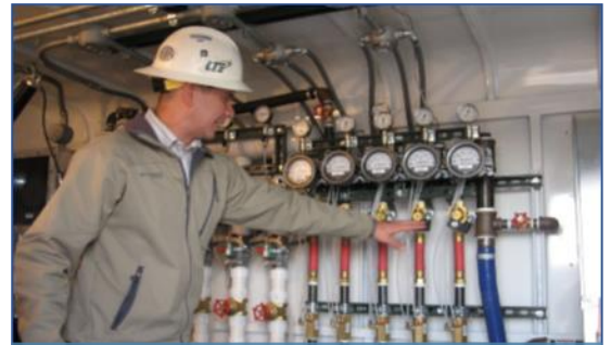
Remediation Design & Implementation
