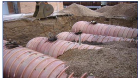
Tank Installation & Removal
